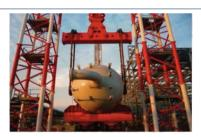
TAILING WITH SPMTs - CRAWLER CRANES - SKID SHOES AND TAILING FRAME
